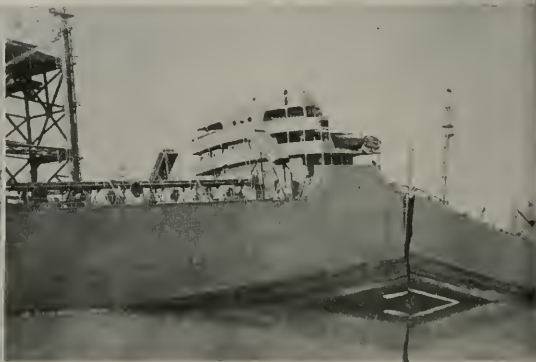
Above left: Adrift 20 miles from stern section, shown here is the bow of the SS Fort Dearborn from which ten crew members were removed by SS St. Johns Victory. The Fort Dearborn broke in two during storm 1100 miles northeast from Honolulu. At right: Broadside view of T-2 tanker Schenectady at builders dock. Fracture is in typical location.
